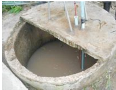
Figure 7: Functioning rope pump Figure 8: Rope pump in the process of repair (replacement of rope, requires replacement of rope, cleaning of the well and replacement of well cover) Sioko village, Choma. Chinyengele village, Magoye.
