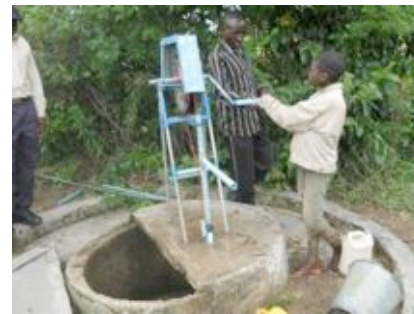
Figure 7: Functioning rope pump Figure 8: Rope pump in the process of repair (replacement of rope, requires replacement of rope, cleaning of the well and replacement of well cover) Sioko village, Choma. Chinyengele village, Magoye.
